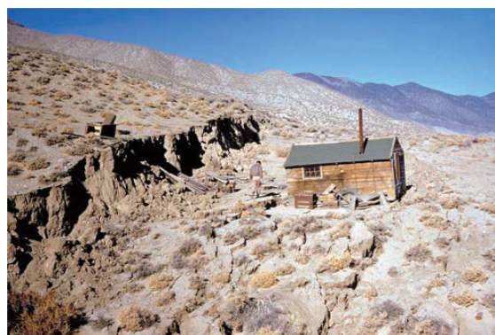
Figure 17. Cabin adjacent to fault that ruptured in the 1954 Dixie Valley earthquake ( M_w 6.9). The photograph was taken on 20 December 1954 by Karl Steinbrugge. The man in the photo is Vincent Bush, a member of the team investigating the earthquake. Source: Karl V. Steinbrugge Collection: S653, National Information Service for Earthquake Engineering (NISEE), University of California, Berkeley. The color version of this figure is available only in the electronic edition.
