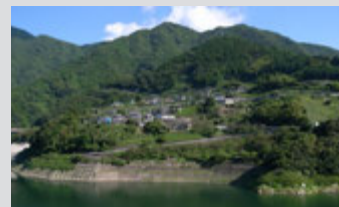
四国山地における典型的な地すべり(地震計による観測斜面) Typical landslide in the Shikoku Mountain (with earthquake observation by means of seismometers)
