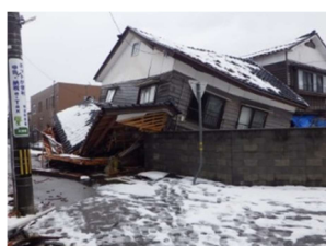
Photo 2-15 Heavily damaged wooden house
