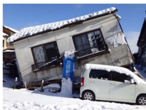
Photo 2-7 Heavily damaged wooden house
