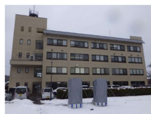
Photo 2-9 Wajima Regional Joint Government Building
