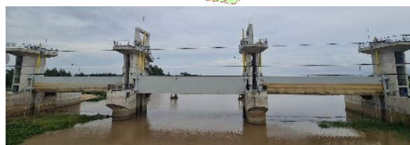
Fig. 2 Locations and a photo of the sluice gate in the field survey from July 31 to August 11, 2023
