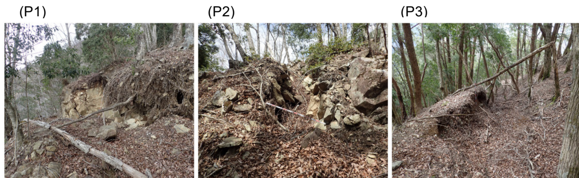
Fig. 15 Photographs of scarps formed above the Uguhara landslide. (P1) View to the north. (P2) View to the north. (P3) View to the south.
