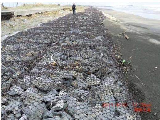
Photo 8 Wave dissipating later to prevent scouring
