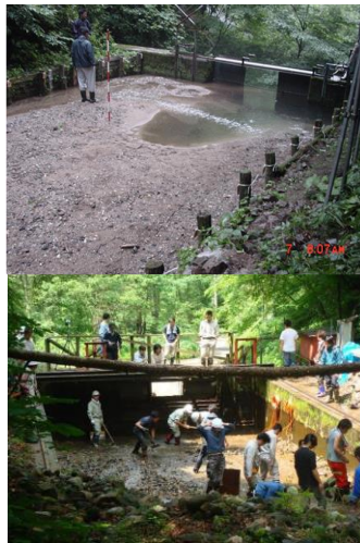
Photo 2 A Check dam in Hiru-dani valley
