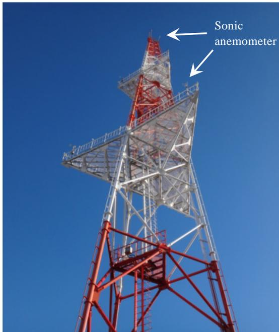
Photo 1 Observation tower in the Ujigawa Open Laboratory. Sonic anemometers at 55 m and 25 m are indicated
