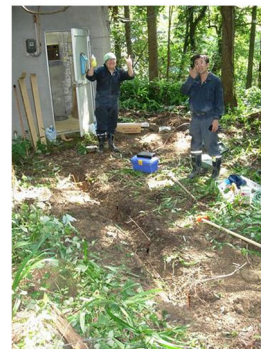
Photo. 7 Class A grounding work
