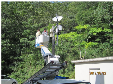
Photo. 8 Antenna installation using aerial work platforms
