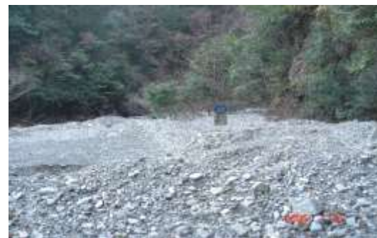
Photo 6 The road was buried with more than 1m debris in Akaba river, Mie pref.
