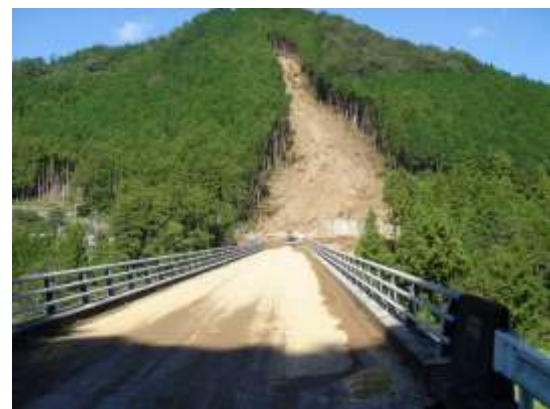
Photo 7 The slope failure flowed to the nearby bridge at Kotaki in Miyagawa river, Mie pref.
