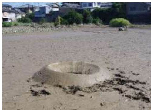
Photo 11 Sand boiling at the farmland beyond the left embankment.
