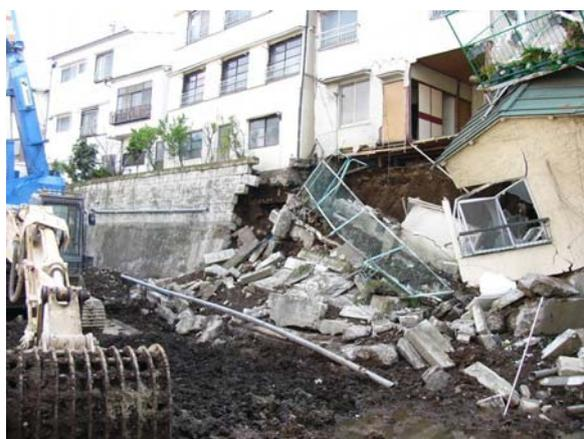
Photo 3 Collapse of small residential fill in Tokyo, 2004
