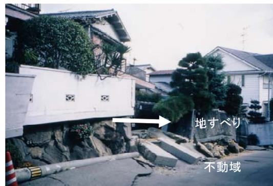
Photo 2 Landslide in residential valley fill in Nishinomiya City, caused by the 1995 earthquake
