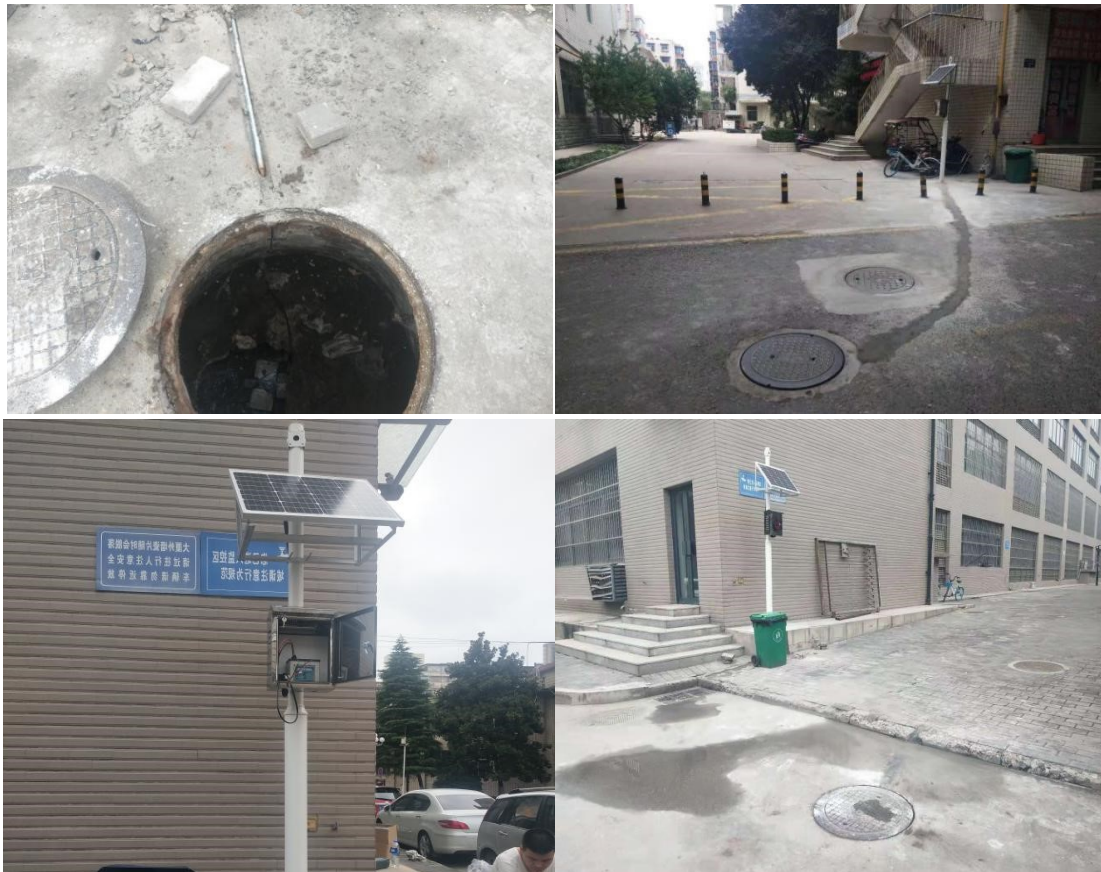
Figure 6 Construction process and effect
