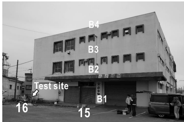
Fig. 11 Temporal earthquake observation stations deployed at the test site and the building [CTOC07]
