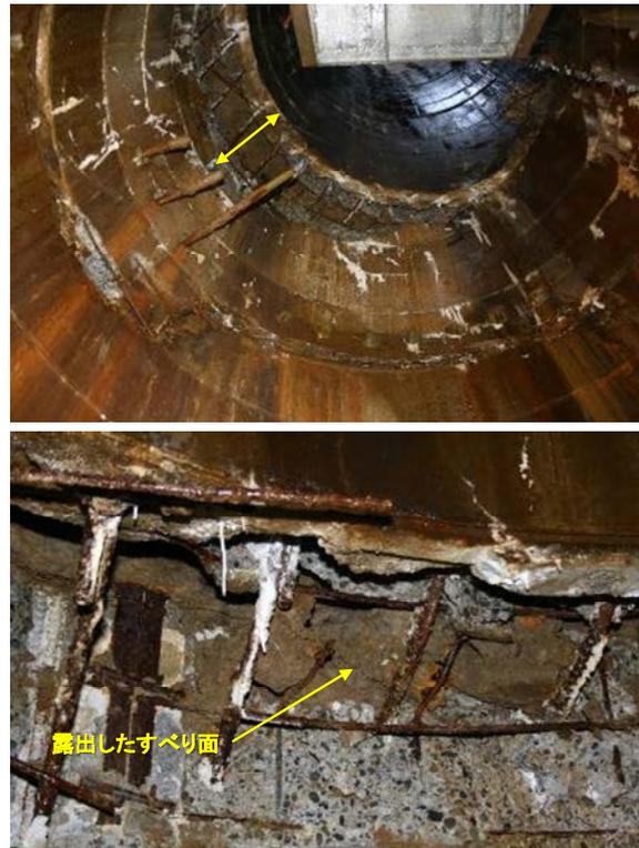
Fig. 13 Destruction of a concrete drainage well due to the displacement of reactivated landslide.
