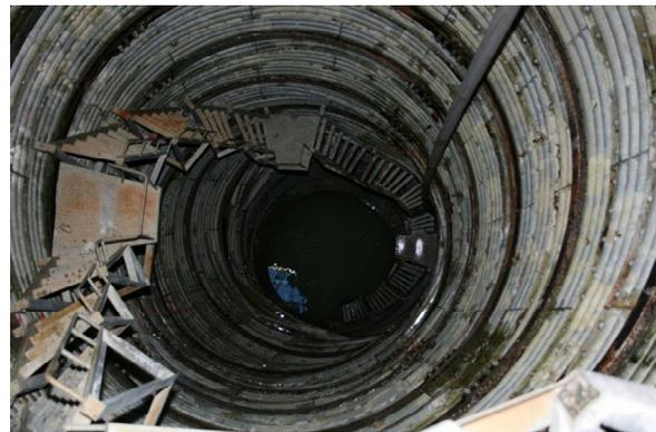
Fig. 15 Deformation and destruction of a drainage well in the accretionary prism landslides.
