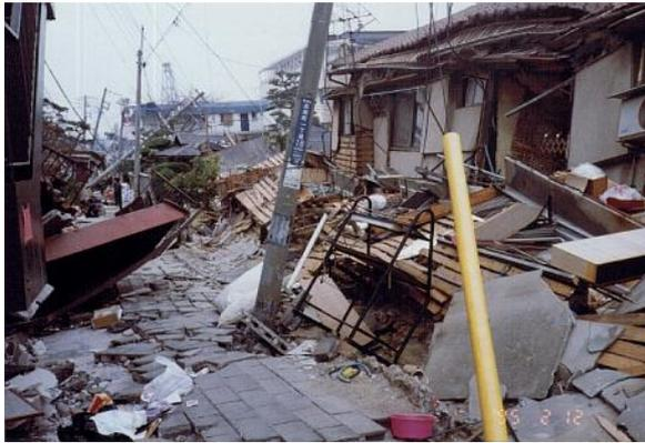
Photo 2 Total road blockage by collapsed wooden houses in Higashinada-Ward 3 weeks after the 1995 Hyogo-ken Nanbu (Kobe) earthquake (Photo by H. Kawase).
