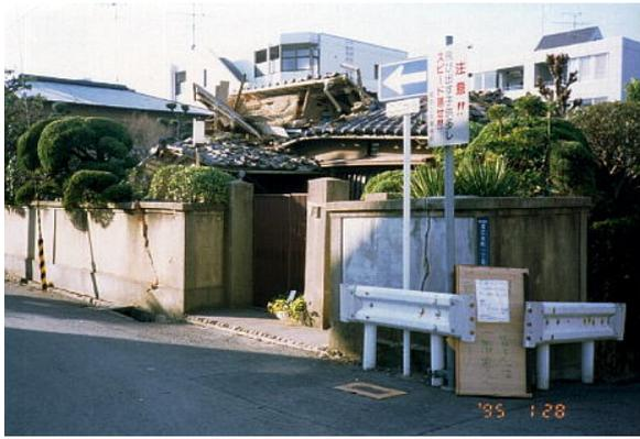
Photo 1 A collapsed wooden house (originally 2-storied) in Higashinada-Ward 11 days after the 1995 Hyogo-ken Nanbu (Kobe) earthquake (Photo by H. Kawase).
