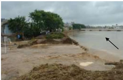
Photo 3 River bank breach at the Asuwa River, Fukui prefecture (Photo: Fukui Shinbun)
