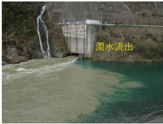
Fig. 4 Turbid water runoff from Sakuma dam (Taken by Takemon)
