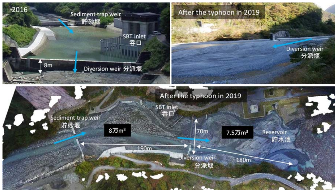
Fig. 5 Sedimentation in the pond and downstream of diversion weir of Koshibu.
