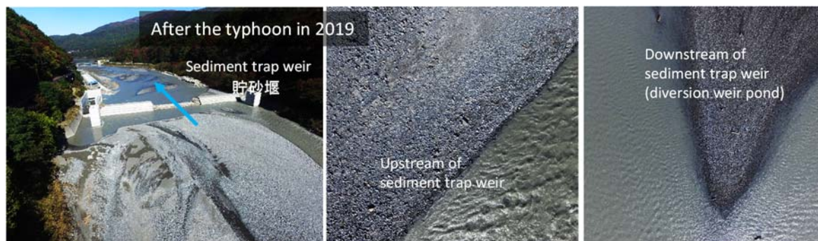
Fig. 6 Sedimentation at the upstream and downstream of sediment trap weir of Miwa
