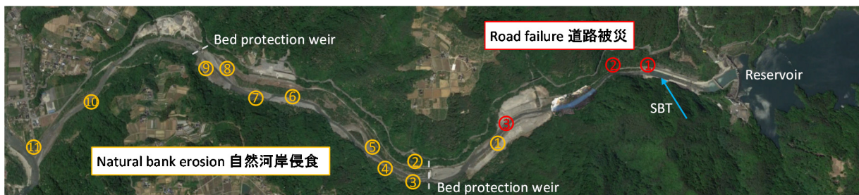
Fig. 4 Location of bank erosion in the downstream of Koshibu Dam in July 2018.
