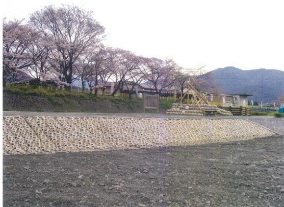
Photo 3 Shore protection using bamboo gabion in the Shimada city (courtesy of Hara Kogumi Co., Ltd.)
