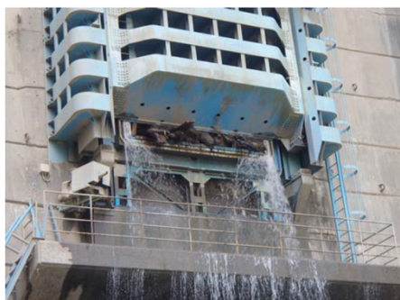
Fig. 1 clogging of outlet of Susobana dam (MLIT, 2018)
