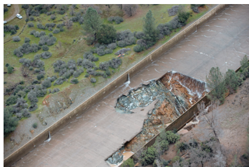
Fig. 2 Oroville dam spillways incident (Matsumoto, 2017)
