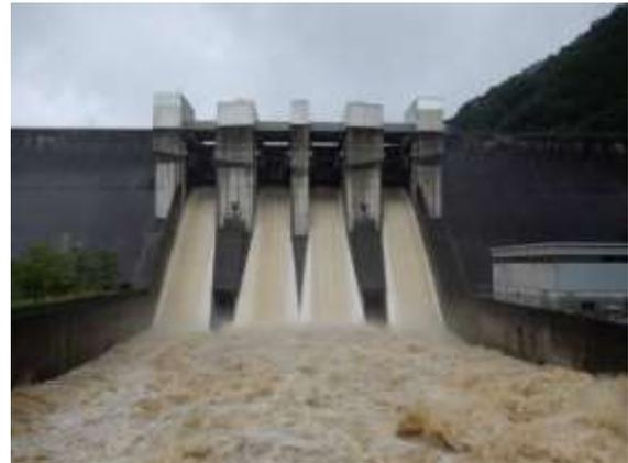
Photo 1 Hiyoshi Dam under the emergency spillway gate operation (provided by Japan Water Agency).
