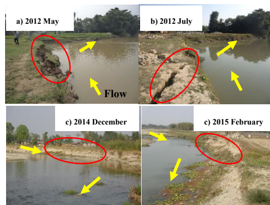
Photo 4: Bank erosion in the study reach; (a & b) Sunsari River and (c & d) Lohandra River
