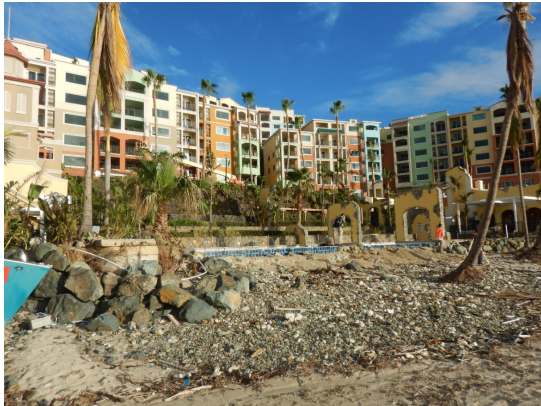
Photo 1: Damage of hotel at the southeast coast in St. Thomas (run-up height is 6 m)
