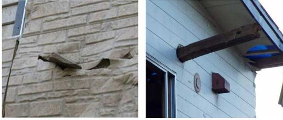
Fig. 1 Damage to the walls of houses by flying debris
