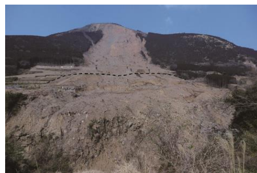
Fig. 4 The landslide on the western slope of the Aso bridge. A dotted line shows the crown of the landslide on the lower slope.
