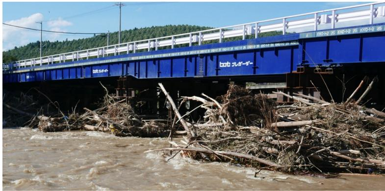
Fig. 9 Accumulation of drift woods on bridges piers of Kiyomi bridge
