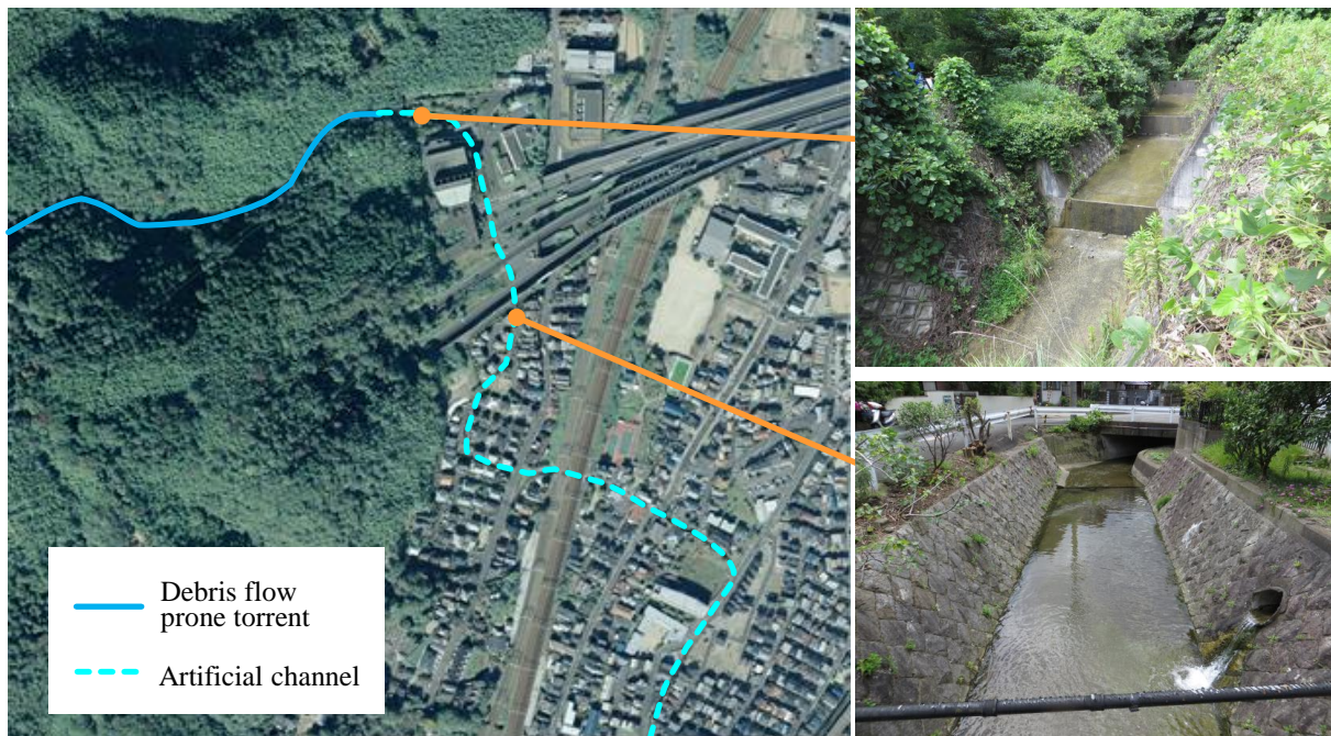
Fig. 2 Flow direction of the artificial channel
