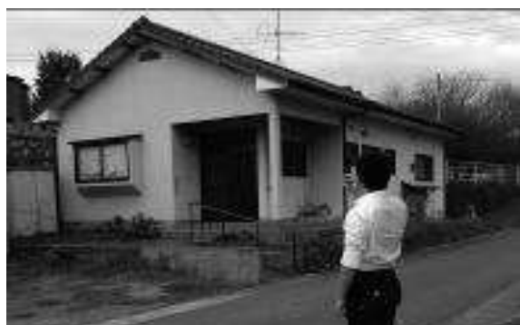
Photo 1 Collection of house façade
