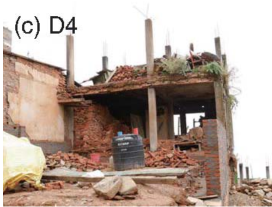
Fig. 4 Photo of buildings with damage levels D2-D4. (a) D2: plasters on the column was fallen down. (b) D3: permanent drift was observed. (c) D4: almost all infill was fallen down.
