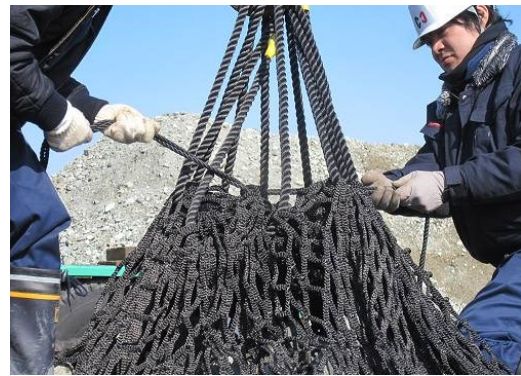
Photo 3 Tightening rope at net-mouth
