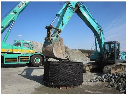
Photo 2 Filling of inner rubble
