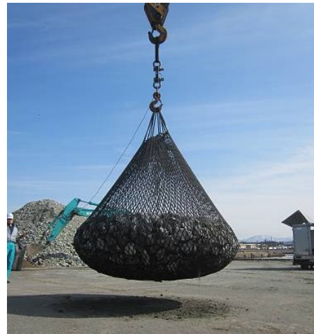
Photo 4 Relocation of net-type unit
