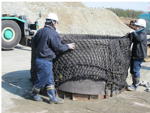
Photo 1 Setting of net inside round flume
