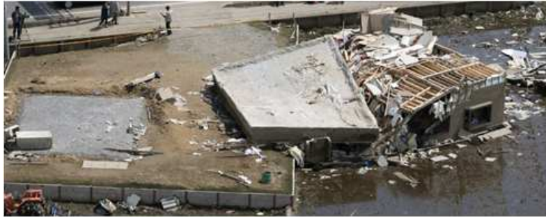
Fig. 8 Turned over wooden house with mat foundation ( photo by Kyodo News )
