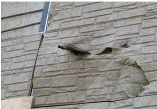
g. Roof tile stuck into a wall
