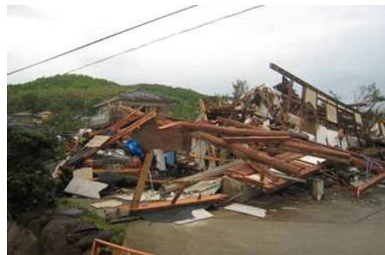
Fig. 13 Collapsed wooden house ( quote from the report of KAKENHI, 2013 )
