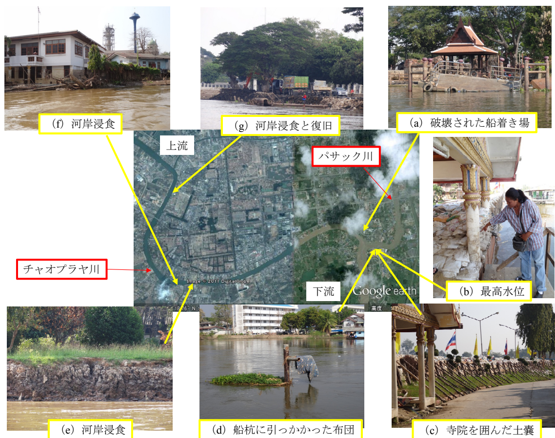
Fig. 3 Flood and bank erosions at world heritage site of Ayutthaya
