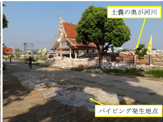
Fig. 5 Piping phenomena
