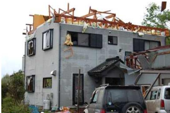
Fig. 12 Blown off roof
