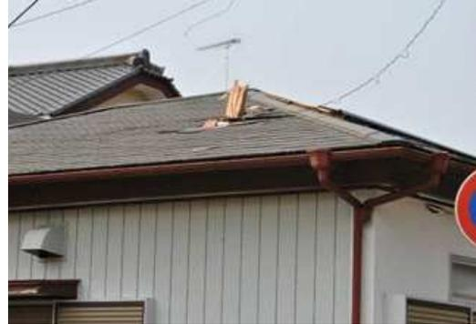
f. Timber stuck into a roof
