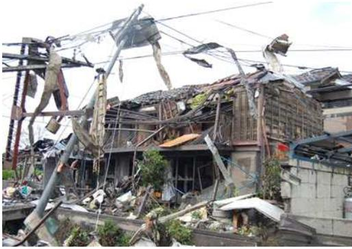
a. Flying debris twining around power lines
