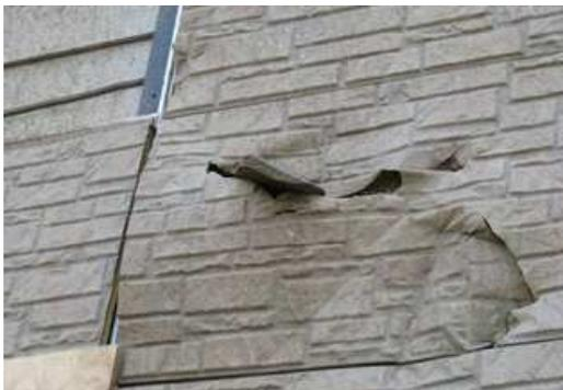
g. Roof tile stuck into a wall
