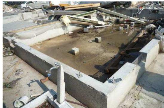
Fig. 7 Foundation of blown off wooden house
