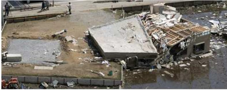
Fig. 8 Turned over wooden house with mat foundation
