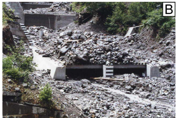
Photo 1 Flat-board debris-flow breaker. (A) After removal of the July 21, 1985 debris-flow deposits and the construction of sidewall reinforcements. (B) Boulder deposits of the July21, 1985 debris flow trapped on the breaker (photo taken July 22, 1985).
