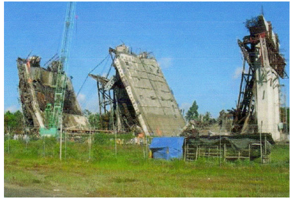
Fig.21 Collapsed concrete girder (Shioi 2011)
