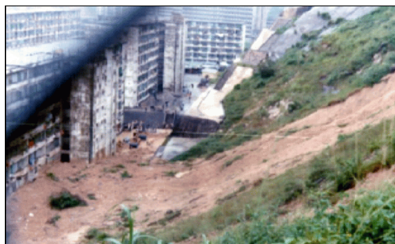
Fig. 1 Sau Mau Ping slope failure: view behind Block 9 (Bolton, 2011)
