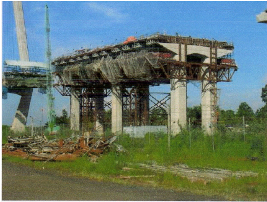
Fig.20 Construction view before collapse (Shioi, 2011)
