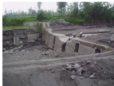
Photo 9(a) Collapse type 1
