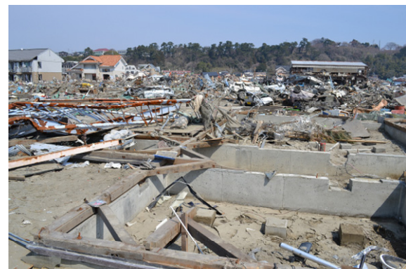
Photo 24 Remained house's foundation
