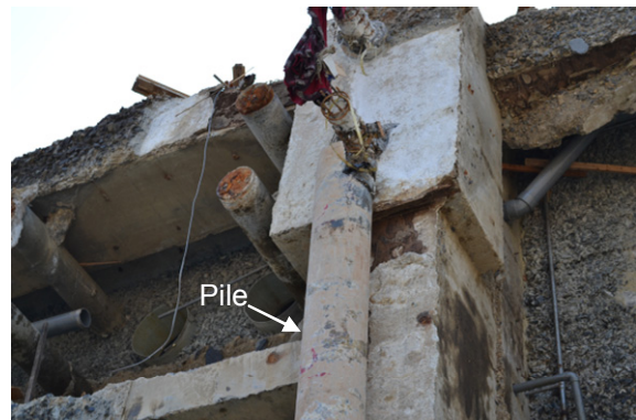
Photo 38 Pile of toppled building F
