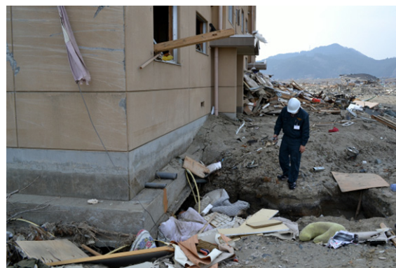
Photo 4 Scour around building B
