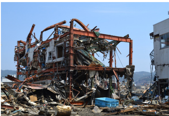
Photo 19 Damage to steel structure
