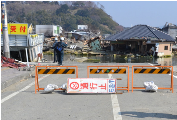
Photo 21 Road washed away by tsunami (Ishinomaki-city)
