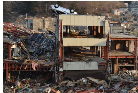
Photo 30 Car on steel 3-story building
