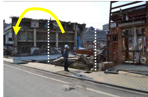
Photo 36 Estimated location of building F
