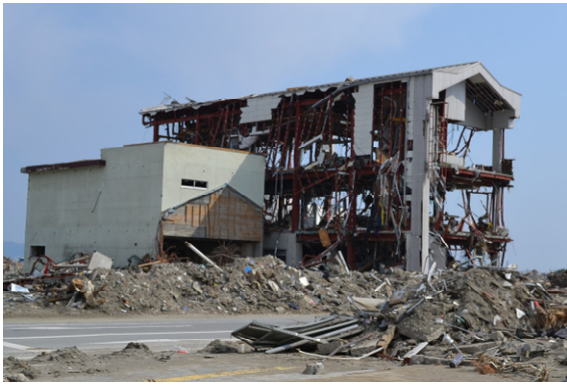
Photo 11 Damage to steel structure
