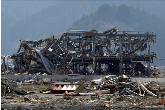
Photo 13 Damage to steel structure
