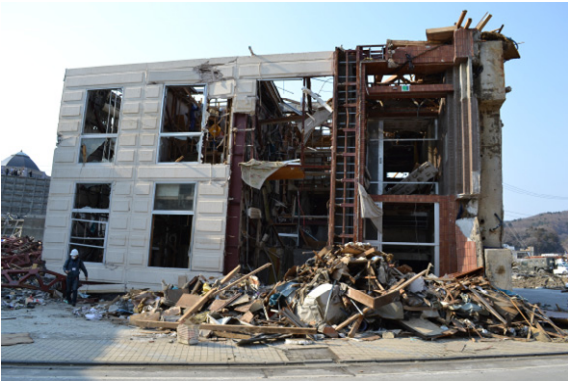
Photo 35 Toppled steel structure 4-story building F
