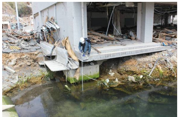
Photo 48 Extensive scour around building J
