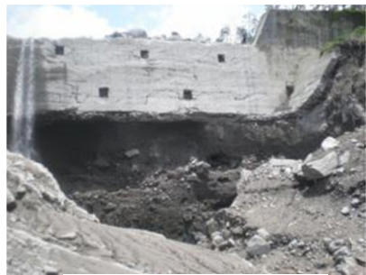
Photo 9(b) Collapse type 2
