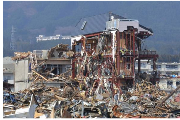
Photo 12 Damage to steel structure
