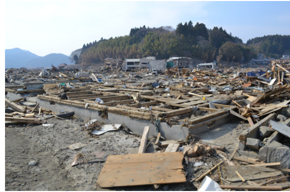
Photo 14 Remained house's foundation
