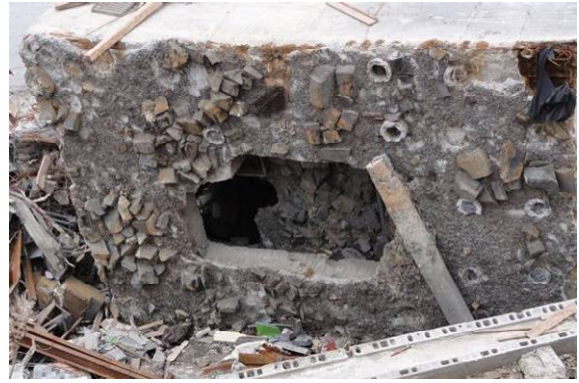
Photo 34 Pile of toppled building E
