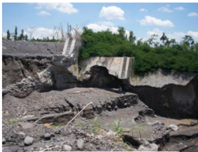
Photo 9(c) Collapse type 3
