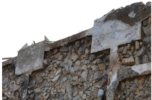
Photo 40 Pile cap of toppled building G
