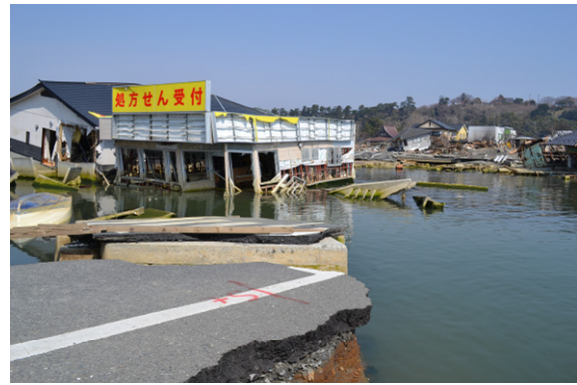
Photo 22 Road washed away by tsunami (Ishinomaki-city)
