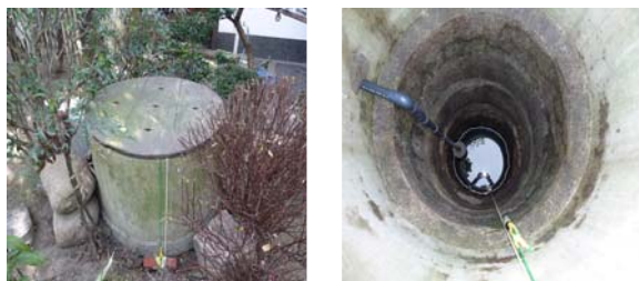
Photo 1 Digging type well
