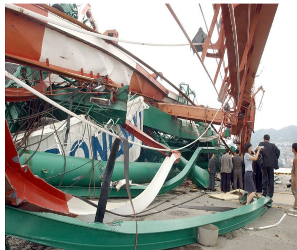
Figure 4 Container cranes in Pusan port destroyed by strong wind during Typhoon MAEMI
