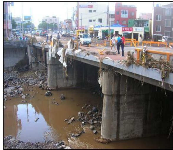
Figure 2 A bridge destroyed during Typhoon RUSA
