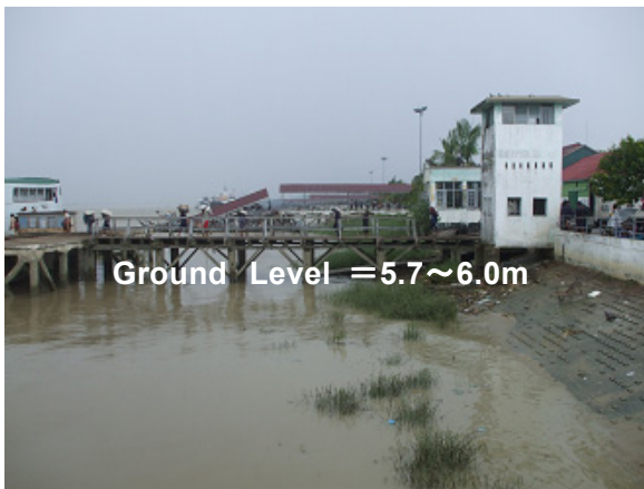
Photo 1 Relation of pier, seawall and road
