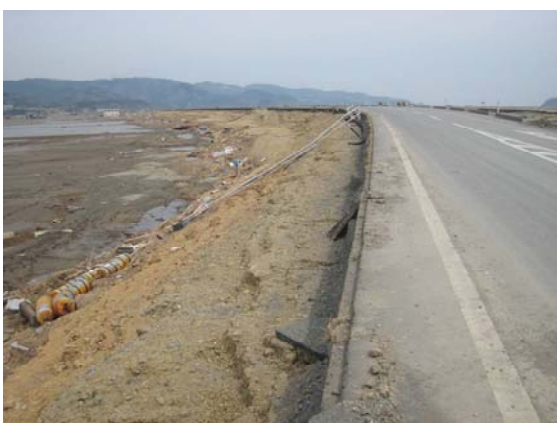
Figure 13 Washed embankment near the Shin Kitakami River
