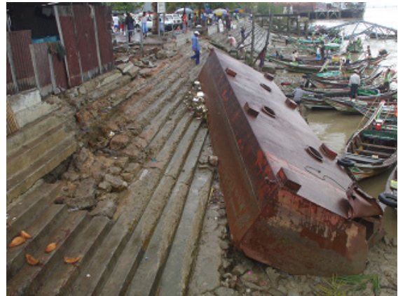
Photo 5 Broken pontoon on seawall
