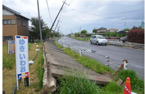
Figure 23 Inclined electric pole and uplifted lids of drain in Hinode cho, Itako city.
