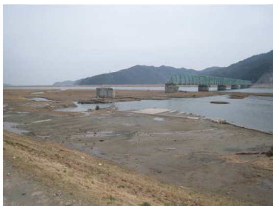
Figure 12 View of the Shin Kitakami bridge.
