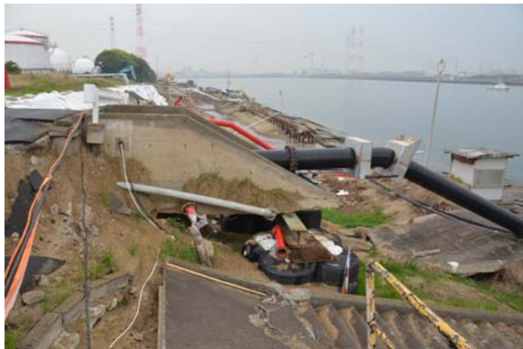
Figure 22 Damaged embankment in Kajima port
