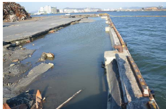
Figure 5 Damaged apron of the Nakajima wharf, I Shinomaki port.
