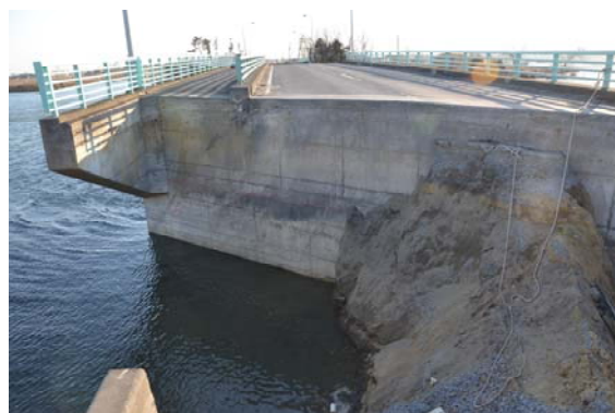
Figure 15 Lost embankment of Jokawa bridge.
