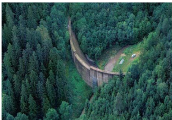
Photo 6 Flood mitigation dam of Ligistbach, Styria, Austria
