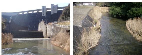
Photo 2 Nunome Dam in the Nunome River and its downstream channel with long riffle
