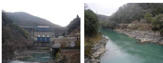
Photo1 Amagase Dam in the Uji River and its downstream channel with long pool
