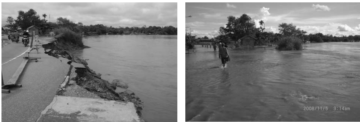
Figure 2 River bank failure and flood at Seluwing Malinau
