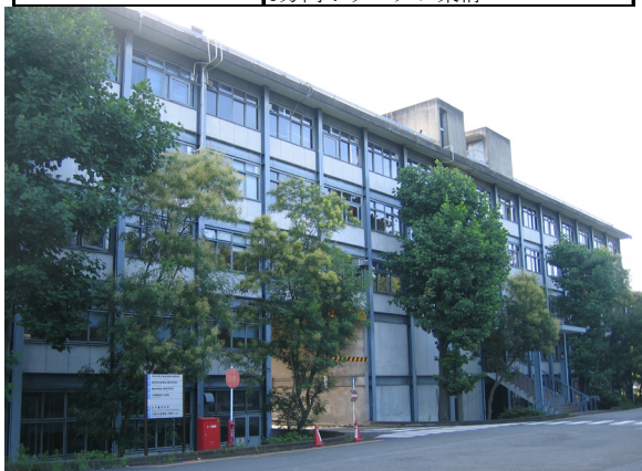
Photo 1 The object building before the reinforcement (Uji campus main research building, east building)
