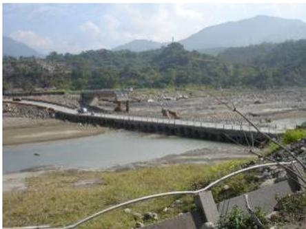
Photo 17 Buckling of steel pipe pile pier
