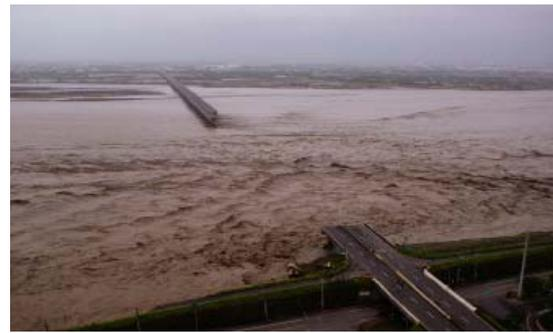
Photo 18 A bridge broken by local scouring
