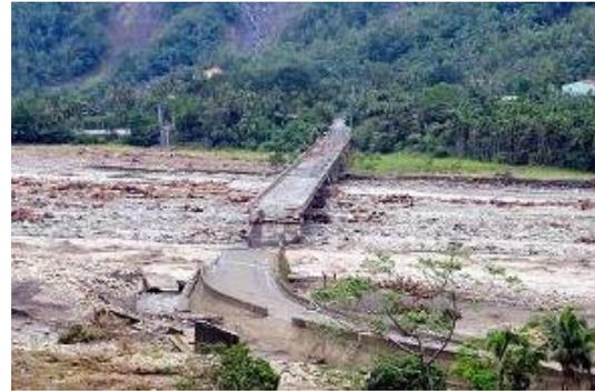
Photo 16 A bridge with broken abutment
