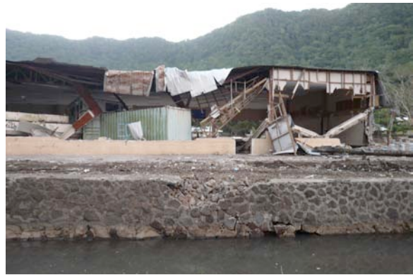
Photo 1 A damaged building in Pago Pago Park.
