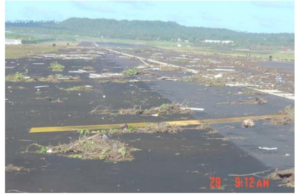
Photo 8 Debris on runway in Tafuna Airport. (Photo provided by Mr. Chris Soti, DPA)
