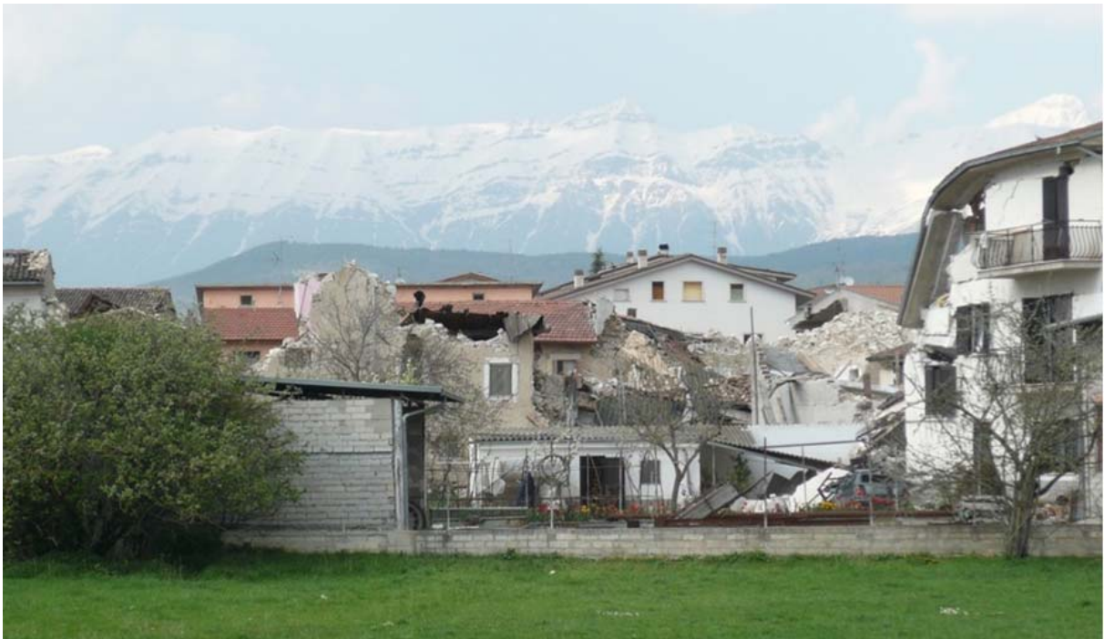
Photo 3. Severe building damage in the village of Onna.
