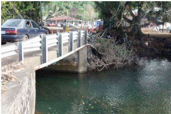
Photo 11 A temporary restored bridge in Leone.
