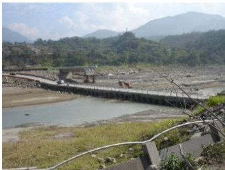
Photo 17 Buckling of steel pipe pile pier
