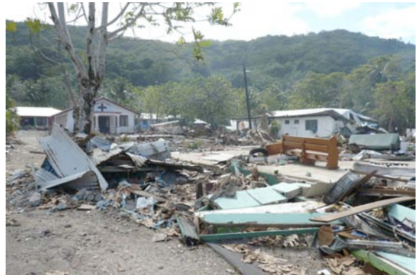
Photo 6 Damages of Amanave.
