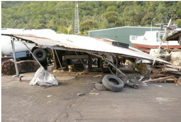
Photo 4 Damages in the vicinity of thermal power plant.
