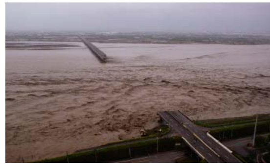
Photo 18 A bridge broken by local scouring
