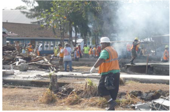
Photo 12 Recovery work in Leone.
