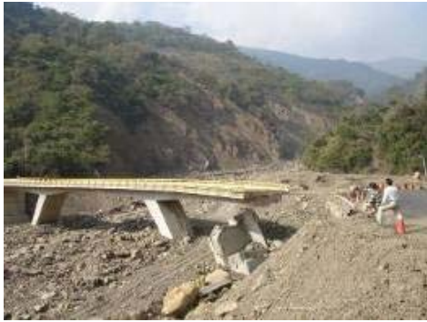
Photo 15 A bridge whose pier is only broken
