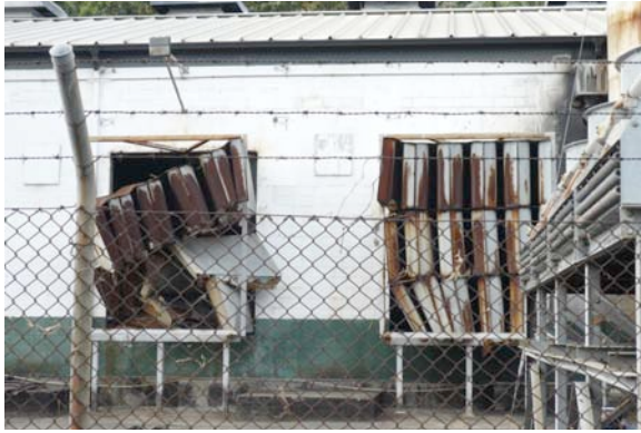
Photo 3 An damaged thermal power plant in Pago Pago.
