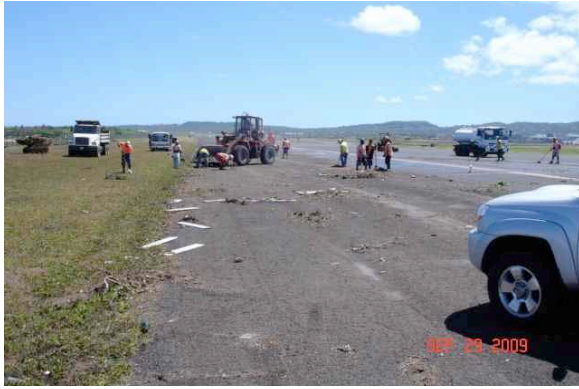
Photo 10 Removing debris from runway in Tafuna Airport. (Photo provided by Mr. Chris Soti, DPA)
