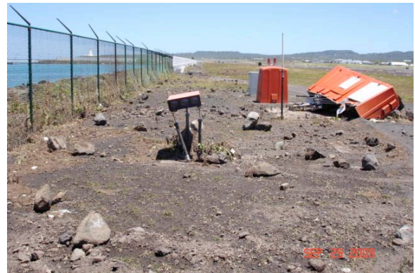
Photo 9 Damaged equipment of Tafuna Airport. (Photo provided by Mr. Chris Soti, DPA)
