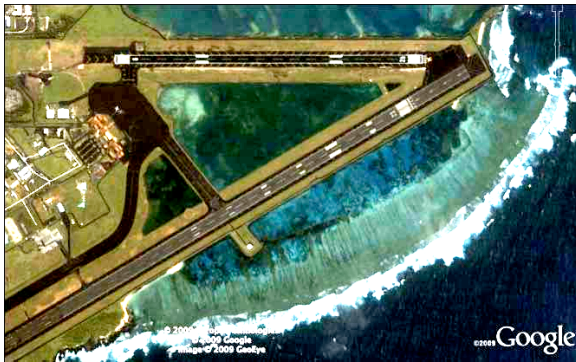
Fig. 4 Satellite imagery of Tafuna International Airport.
