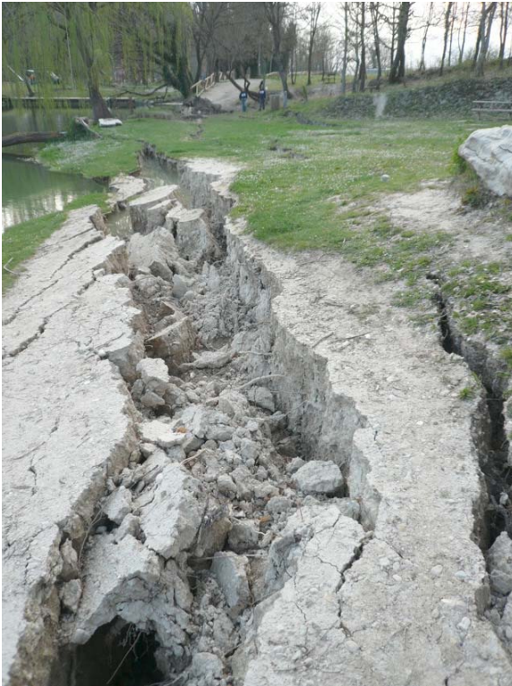
Photo 5. Ground cracking due to subsidence at Lake Sinizzo.
