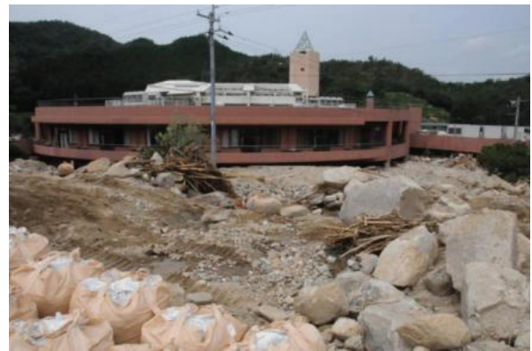
Fig. 5 Photo of the special elderly nursing home damaged by debris flow. The mountain-side rooms on the first floor were filled with the sands.
