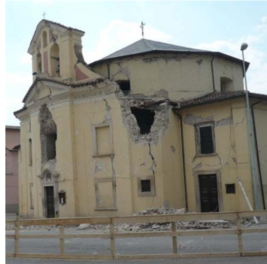
Photo 1. Damage to an old church in Paganica
