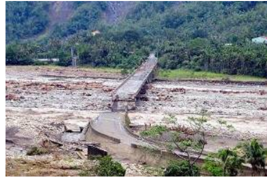
Photo 16 A bridge with broken abutment
