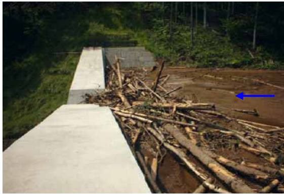
Fig. 3 Debris flow and driftwood captured by sabo dam at Tenryu River, Okaya, Nagano Pref., Japan, 2006 (Source: Sabo Department, MLIT, Japan)
