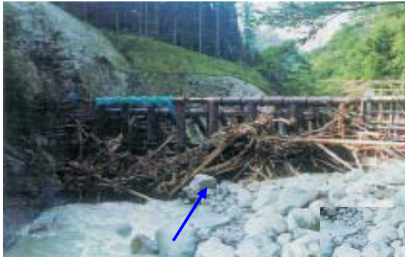
Fig. 2 Debris flow and driftwood captured by grid dam at Agi River, Nakatsugawa, Gifu Pref., Japan, 2000 (Source: Sabo Department, MLIT, Japan)
