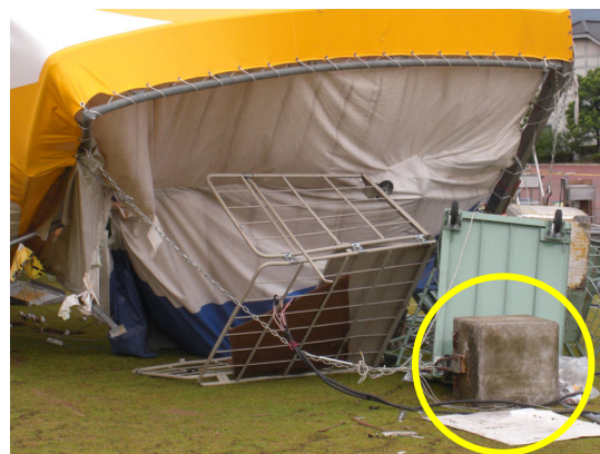
Photo 1 A concrete mass of 300kg to resist wind induces lift.
