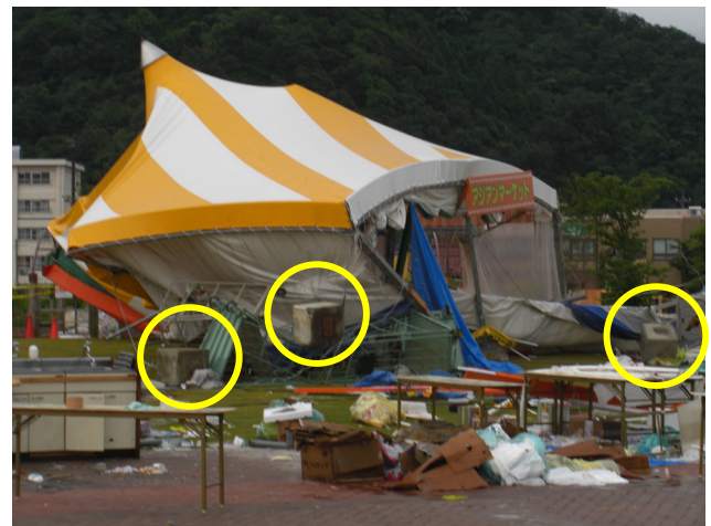
Photo 2 Failure of the large tent structure due to severe gusty wind (circles indicate concrete mass of 300kg). A man was killed by the impact of failed Tent.
