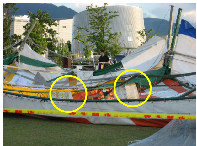
Photo 3 Turned inside out tents together with concrete weights due to severe gusty wind.
