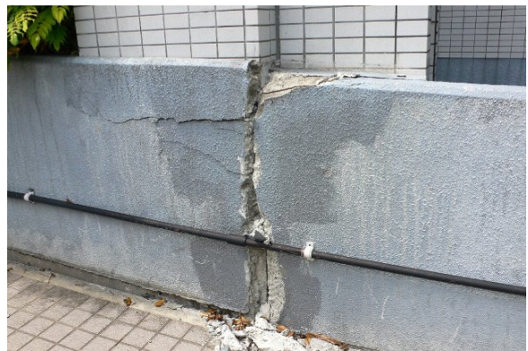
Photo 7 Damage of the non-structural element (walls) near the station IWTH25
