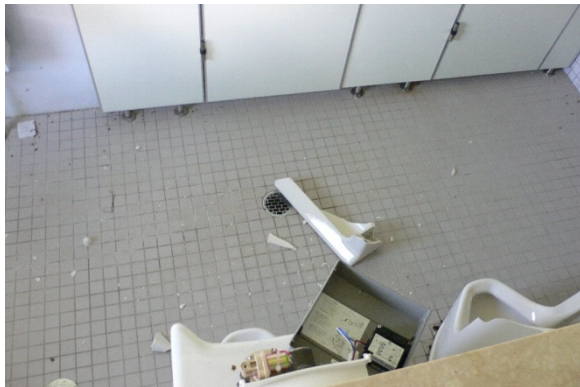
Photo 5 Damage of the non-structural element (ceramics) near the station IWTH25
