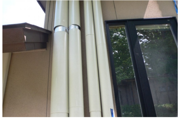
Photo 6 Damage of the non-structural element (pipes) near the station IWTH25
