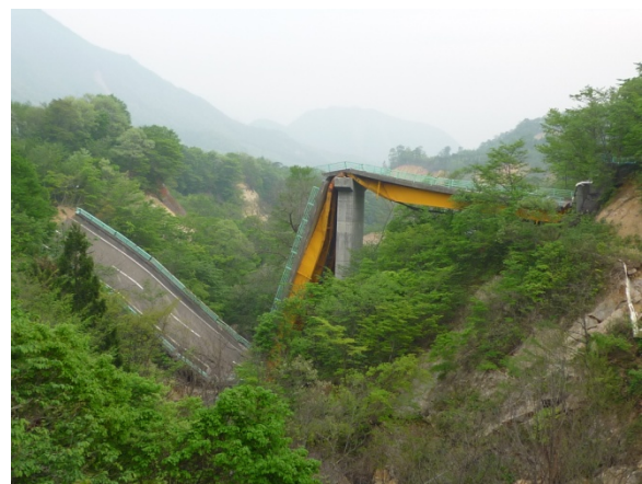
Photo 1 Collapse of the Maturube bridge
