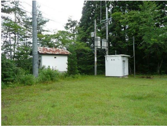
Photo 8 KiK-net station AKTH04 is located on top of the hill
