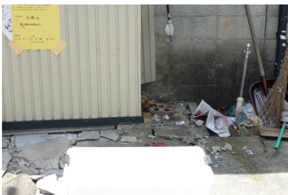
Photo 3 A severely collapsed house near the station IWTH25
